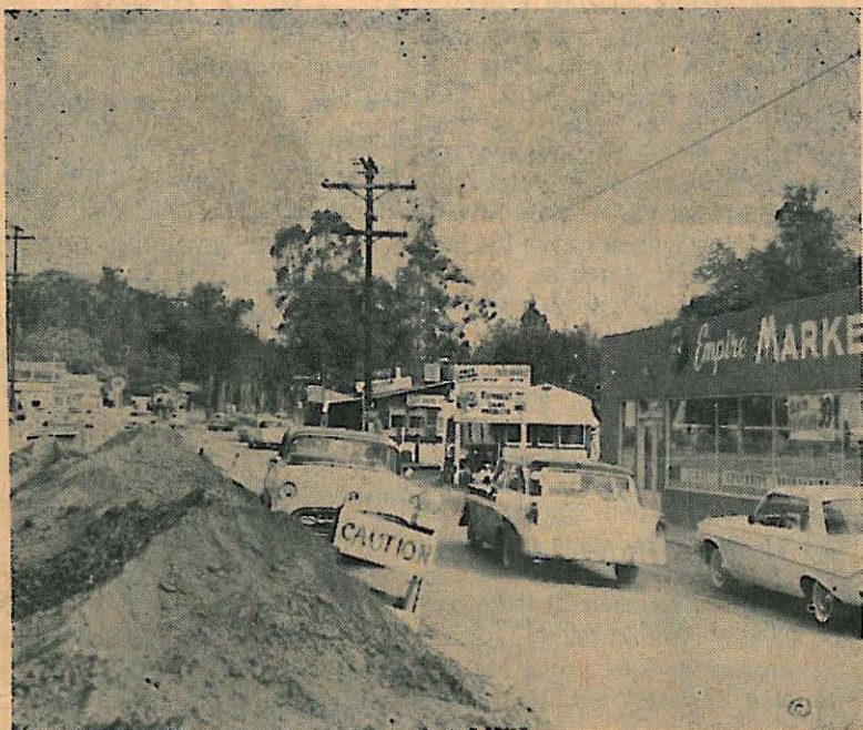
Pipeline Installation Continues East
